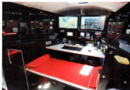
AAL has duplicate nav stations with redundancy built into all the systems.
